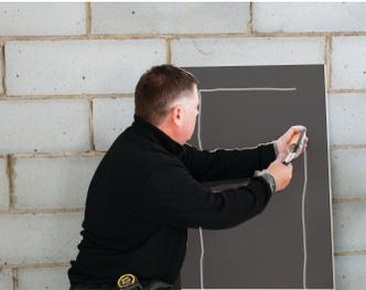
**3 Timber Surfaces.** Fix boards to timber surfaces using STS mega adhesive, plus 6 screws and washers.
