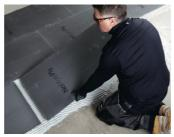
**2 Solid Surfaces.** Fix boards to solid surfaces in a brick bond pattern using flexible tile adhesive.
