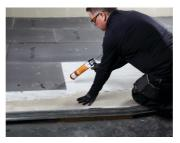
**4** Always seal the joints using STS mega adhesive to ensure a waterproof finish.
