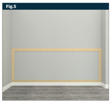
Offer remaining upright strips between top and bottom strips and space them according to figure worked out in Fig 4 i.e example 326.5mm between strips. Check using spirit level. Secure with nail gun **(Fig 6)**.
