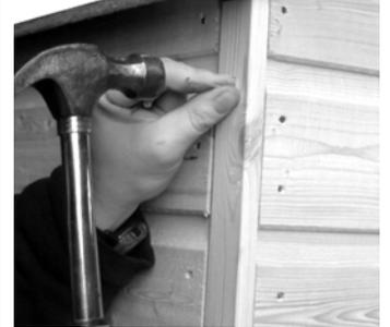
1. Secure remaining three cover strips in position where the panels meet using 3 x 40 mm nails per strip.
