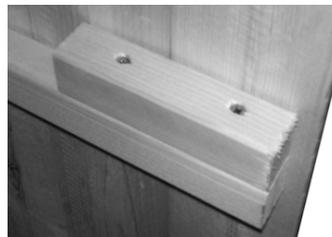
6. Pre drill two holes in pad bolt fixing block. Place block to the top side of the central bracing framework on the back of the door and secure using 2 x 60 mm screws.
