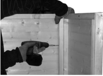
4. Place back panel and a side panel at one corner of the floor ensuring the cladding has overhung the floor. Secure together from the inside using 3 x 60 mm screws. **THE SIDE PANELS EXTEND FROM FLOOR EDGE TO FLOOR EDGE. THE PANELS AT THE BACK AND FRONT SCREW TO AND FIT INSIDE THE SIDE PANELS.**
