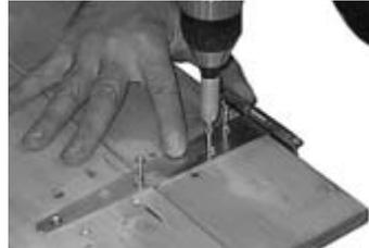
3. Lay door down onto a flat level surface. Check which side of the door the hinges are to be fitted. The side where the bracing does not extend to the edge of the boarding is the hinge side.
