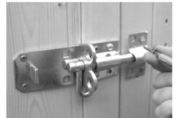
1. Place pad bolt on the outside of the door directly over the horizontal brace. Ensure the edge is flush with the edge of the door. Secure to door using 4 x 25 mm screws using the round holes only.
