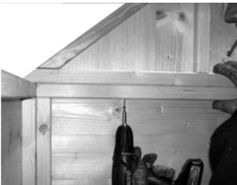
1. Place one gable on top of back panel ensuring the outer edges are flush with shiplap of side panels. Secure from underneath panel framework into gable using 2 x 60 mm screws.
