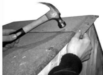
3. Place roof panel, with felt on all sides fixed, into position flush with front and back of building. Secure through roof panel into gable framework using 3 x long felt nails per gable edge and 2 x long felt nails into side wall.
