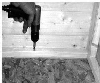
1. Secure wall panels to the floor on the inside of the building using 2 x 60 mm screws for back and side panels and 1 x 60 mm screw for wing panel, preferably into floor bearer.
