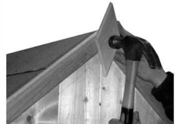
1. Secure the four fascia boards to gable ends using 3 x 40 mm nails per fascia piece.
