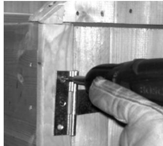
5. Place door into aperture, check door is square and even all the way round and secure in place using 3 x 25 mm screws per hinge.
