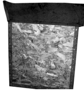
2. Place other roof panel onto the remaining piece of felt, allowing an overhang of approx. 45 mm on three sides and an approx. overhang of 200 mm on the fourth side. Fold felt over onto roof panel, except for the side with the approx. 200 mm overhang, and secure in place using felt nails.
