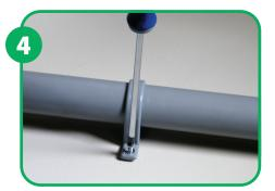
All pipes must be supported both vertically and horizontally.
