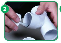
Apply solvent cement to the outside of the pipe and inside of the socket. Leave for 2 or 3 seconds for the cement to work on the plastic.
