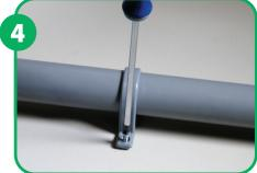
All pipes must be supported both vertically and horizontally.
