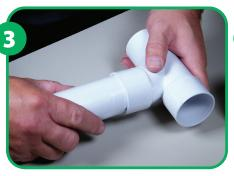
In one swift movement, push the pipe into the socket. Allow 5 minutes for the solvent to bond before handling.
