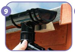
Downpipe installation starts at the outlet. If an offset is required use two Offset Bends with or without a short piece of pipe.
