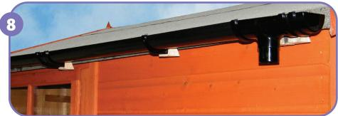
Use a Union Bracket or Angle to join to next gutter length in order to build up a gutter run. Use a Stopend to complete the run.
