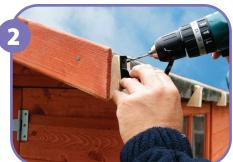
Fix a fascia bracket at the furthest point from the outlet.
