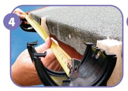
Fascia Brackets should be spaced at a maximum of 500mm apart on straight gutter runs.
