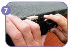
Working from the Running Outlet insert the back edge of the gutter under the retaining clip.
