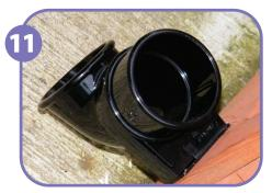
A supporting Pipe Clip should be used on Shoes, Bends and Connectors, where necessary.
