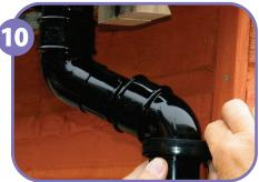
Support downpipes below offset and at maximum intervals of 1 metre.
