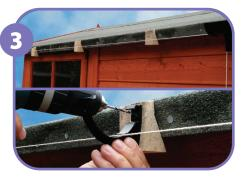
Use a string line between the bracket and the outlet to determine a straight line (if fitting to a fall, 1:350 is recommended).
