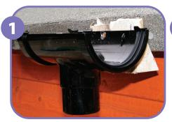
Establish the position of the running outlet and fix the wooden block to the shed.
