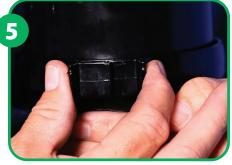
Squeeze the clips at the back together to secure the Strap on Boss to the soil pipe.
