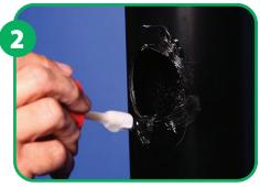
Solvent weld around the hole and the flange of the Strap on Boss.
