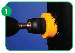
Cut a 54mm hole into the soil pipe.
