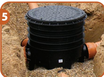
15 Backfill with pea shingle up to the crown of the pipework, and then backfill using the dug out soil.
