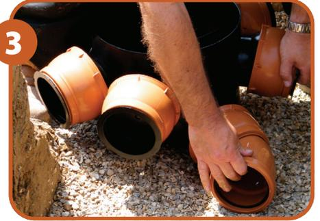
**3** Plan out where the major fittings will sit. Align the inspection chamber so that the flow of water is maintained through the main channel.
