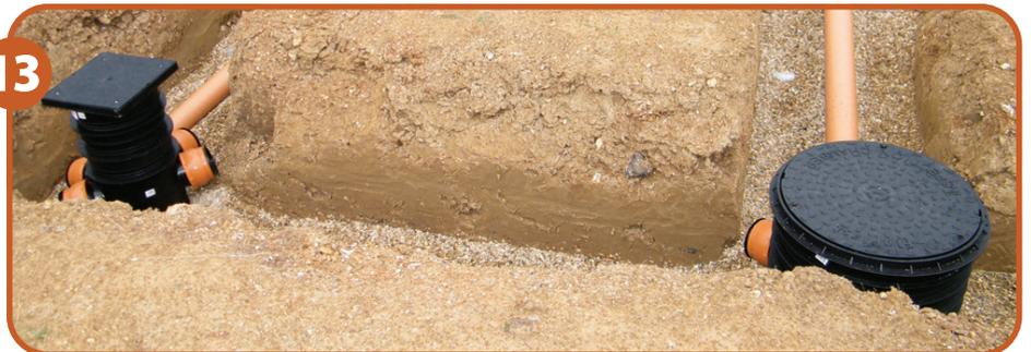
13 Mini Access Chambers (MAC) can be added up to a maximum height of 600mm. Large Inspection Chambers (LIC) can be up to 1.2m in height with the standard 450mm frame and lid. They can be added up to 3m using a 350mm reduced access frame and lid.
