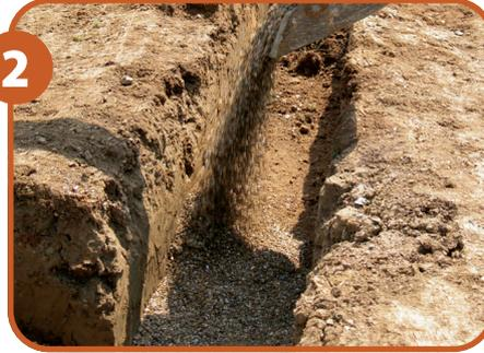
**2** To ensure the pipe is supported correctly, drop in pea shingle to form the pipe bed.
