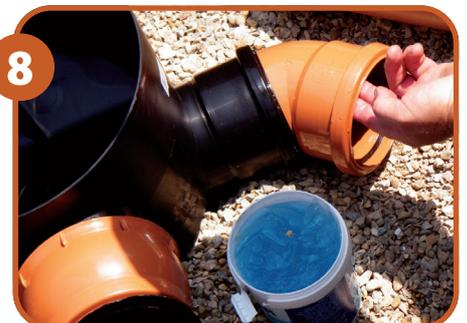
**8** Join the first piece of pipe using a spray or gel silicone lubricant on the seal to ease fitting. Repeat the previous procedure for all the remaining fittings.
