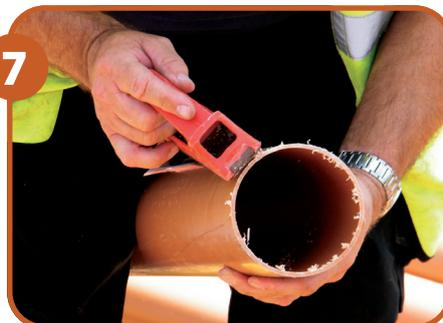
**7** Ensure all cut lengths of pipe are chamfered to roughly a 45° angle.
