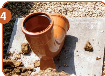
**4** If fitting to a vertical soil and ventilation pipe, it is important to place a solid support under the long radius rest bend.
