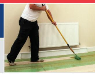
SETCRETE™ ACRYLIC PRIMER prevents unacceptably rapid drying of Coverage SETCRETE™ FLOOR LEVELLING COMPOUNDS over absorbent subfloors, and promotes adhesion to non-absorbent surfaces. It is suitable for use over normal underfloor heating installations and is coloured green to provide the user with visual control of coverage uniformity.
