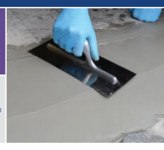
**SETCRETE<sup>™</sup> CONCRETE REPAIR** is an easy to use, single component, Polymer Cement Concrete (PCC) mortar for the non-structural repair of damaged or worn concrete. It is suitable for use on both internal and external applications and can be applied to horizontal and vertical concrete surfaces.
