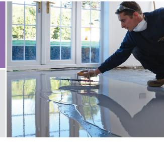
**SETCRETE™ LATEX** is suitable for use over a wide range of absorbent subfloor types including sand/cement screed and concrete. It is also suitable for use over non-absorbent subfloors such as ceramics, granolithic, terrazzo, epoxy and polyurethane resins and quarry tiles, providing they are sound, well adhered and suitably prepared.
