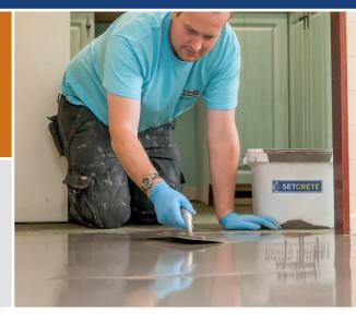
SETCRETE<sup>™</sup> HIGH PERFORMANCE is suitable for use over a wide range of absorbent subfloor types including plywood, sand/cement screed and concrete. It is also suitable for use over non-absorbent subfloors such as granolithic, terrazzo, epoxy and polyurethane resins, ceramic and quarry tiles. The versatility of the product allows for application between 2–10mm on plywood and up to 15mm on concrete. Wearing surfaces should be a minimum of 5mm thickness.
