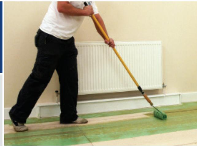
**SETCRETE™ ACRYLIC PRIMER** prevents unacceptably rapid drying of SETCRETE™ FLOOR LEVELLING COMPOUNDS over absorbent subfloors, and promotes adhesion to non-absorbent surfaces. It is suitable for use over normal underfloor heating installations and is coloured green to provide the user with visual control of coverage uniformity.
