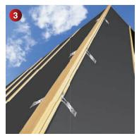
Place the first ridge batten in the batten bracket, and nail through the holes provided in the flange. Build up the ridge batten to the required height by adding one or two more battens, nailing each to the previous batten to ensure it's adequately secured in place.
