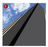
Install the underlay and battens as normal, leaving the underlay 5-30mm short of the ridge on both side. Do not fix the top tiling batten at this stage.
