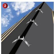
Place the ridge batten brackets across the apex of the roof, and nail to the rafters on both sides of the roof, using the nails provided. (Each kit contains enough batten brackets to fix at 450 and 600mm centres.) Install the top tiling batten as normal, leaving a 10mm gap before the ridge batten.
