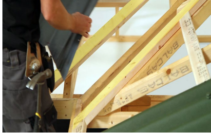
Valley support structure The support structure to the valley is constructed by first fixing trimming battens to the purlins, and lining with valley boards to provide a 7.5cm gutter depth.
