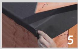
Re-install any existing timber barge boards to help secure the membrane perimeter. Replace if rotten.
