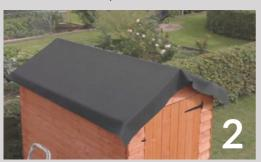
Relax the rubber membrane by laying it in position on the roof for 20 minutes. Fold membrane back to centre of roof for adhesive when ready.
