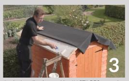
Apply the adhesive working IN STAGES towards the edge of the roof. Roll membrane onto adhesive whilst wet. Re-apply more if necessary.
