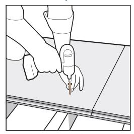
Secure with 12 x 38mm STS Drill Tip screws, placed a minimum of 12mm from the square edge and 5mm from the side of the joist. Ensure screws are placed a minimum distance of 25mm from the tongue and groove edge.
