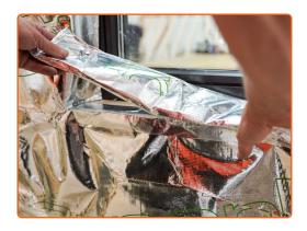
You should then cut two additional strips of insulation to fit the top and bottom of the reveal. Measure the internal width and depth of the window reveal, this will provide the dimensions of these additional strips. Once cut to an appropriate size, these should be sealed on all edges using SuperFOIL Multifoil tape in accordance with the guidance provided on page 9.
