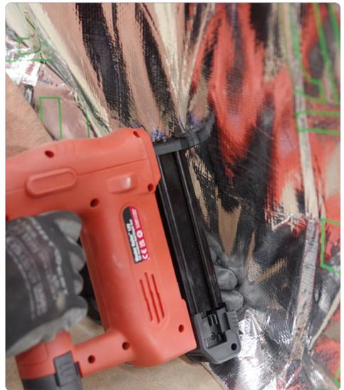
It's important to seal all joints, tears and cuts using SuperFOIL Multifoil tape to ensure an airtight finish. This will help prevent air leakage, improve the thermal performance of the insulation, and maintain condensation control.
