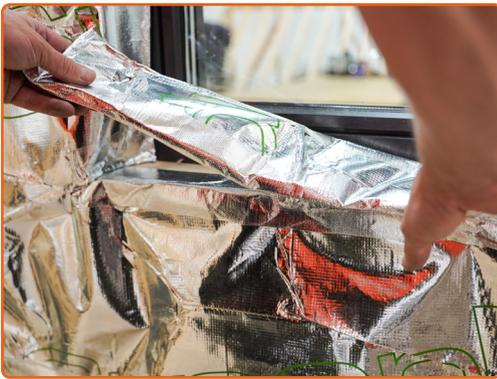
You should then cut two additional strips of insulation to fit the top and bottom of the reveal. Measure the internal width and depth of the window reveal, this will provide the dimensions of these additional strips. Once cut to an appropriate size, these should be sealed on all edges using SuperFOIL Multifoil tape in accordance with the guidance provided on page 9.
