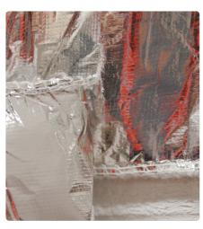
When installing the next layer of the SuperFOIL be sure to overlap the previous layer by at least 50mm. Secure the SuperFOIL to the battens with 14mm staples at no more than 300mm intervals. Again when finishing at a wall, ceiling, floor and any window and door openings, please leave 50mm overlap to create a seal under the perimeter battens.
