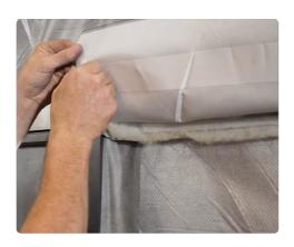
Once you have secured a run of SuperFOIL, you should seal it to the preceding run before beginning the next run.
