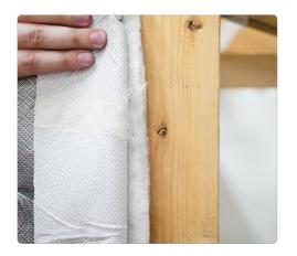
The SuperFOIL should be installed horizontally against the battens with the breathable membrane surface facing away from the wall and the perforated foil side facing toward the wall.
