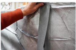
If you finish a roll of insulation in the middle of the wall, turn back the breathable membrane top layer, and trim the revealed insulation layers back to the centre of the last covered batten. As you do, take care not to cut or otherwise damage the breathable membrane top layer.
