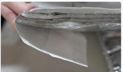
Before installing the insulation, you'll need to prepare the first run of SuperFOIL. To do this, you should first measure the length of the wall being insulated and cut an appropriate length of insulation to fit the wall. This is the first run of insulation.
