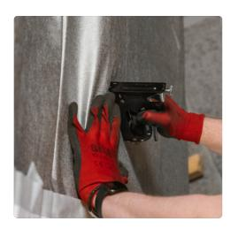
To fix the product, you'll need to staple one end of the run to the battens at the edge of the wall and work along the length of the run, securing the insulation as you go. When securing the product, you should remove excess slack by applying gentle tension before stapling.
