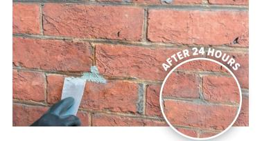
**Stormdry**<sup>®</sup> **XR-Mortar** cures by evaporation of moisture. In cold and damp conditions this drying process can be slowed, especially when applied in thick layers. For thick applications it may be necessary to apply the mortar in two layers to achieve an even cure. When applying the second coat push the mortar into the first coat for a good bond.
