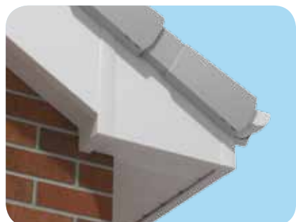
Gable end showing corner trims
