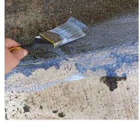
We recommend a small discreet area approximately 1m² is treated with the SEAL IT LIQUID MEMBRANE prior to applying to the full surface area for the purpose of identifying any adverse reaction between product and the substrate.
