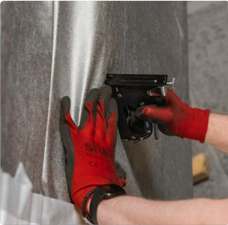
To fix the product, you'll need to staple one end of the run to the battens at the edge of the wall and work along the length of the run, securing the insulation as you go. When securing the product, you should remove excess slack by applying gentle tension before stapling.
