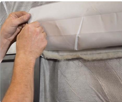
Once you have secured a run of SuperFOIL, you should seal it to the preceding run before beginning the next run.
