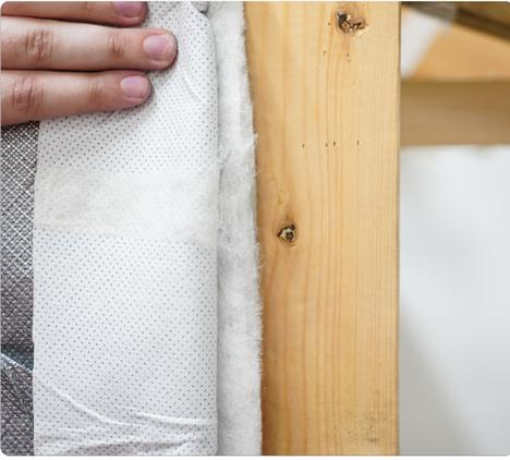
The SuperFOIL should be installed horizontally against the battens with the breathable membrane surface facing away from the wall and the perforated foil side facing toward the wall.
