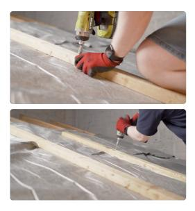
We highly recommend using counter battens alongside any SuperFOIL insulation product.
