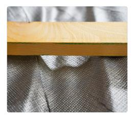
Alternatively, if you decide to apply the tile battens directly to the insulation layer, you need to ensure that the product is draped between the rafters to create a 10mm gap (at least) under the tile battens to allow water run-off.
