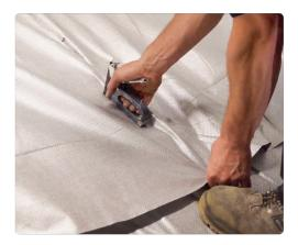
To enhance airtightness, it is important to seal the 100mm overlap to the previously installed roll.
