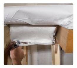
At the wall plate you should ensure that the insulation layers (beneath the breathable membrane top layer) overlap it slightly.
