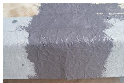
Double reinforced trim joint
