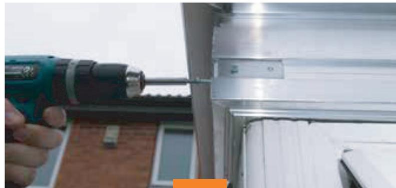
CONTINUE LOCATING THE RING BEAM USING THE INTERNAL AND EXTERNAL BRACKETS AND SELF-DRILL SCREWS
