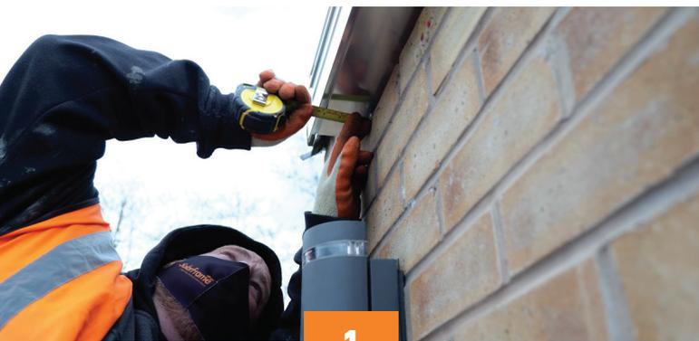
ALIGN THE LOCATING NIB WITH THE FRONT EDGE OF THE WALL/FRAMES AND MEASURE TO ENSURE EACH END OF THE RING BEAM IS THE SAME DISTANCE FROM THE BRICK OR FRAMES
