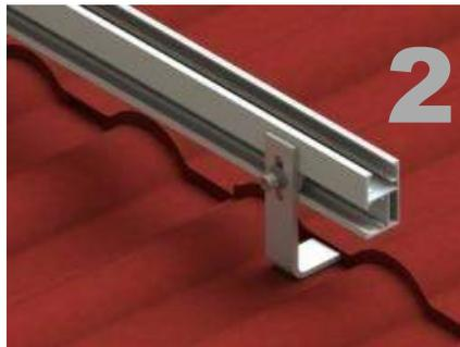
Fix the GS rail to the roof hook with GS Nut.
