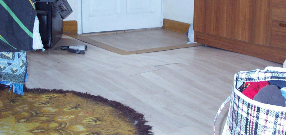
Bulging / distortions
