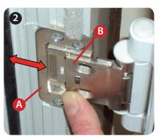
Carefully slide the door away from the frame plates.
