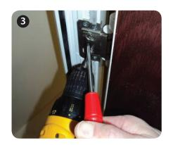
Secure the screws in the side plate.
