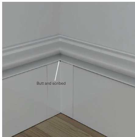
Internal Corners: Capping should be butt and scribed
