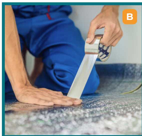
Tape all floor insulation joints.
