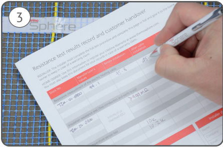
Make sure to record the results. Repeat steps 1-3 for Mesh heating mat insulation test.
