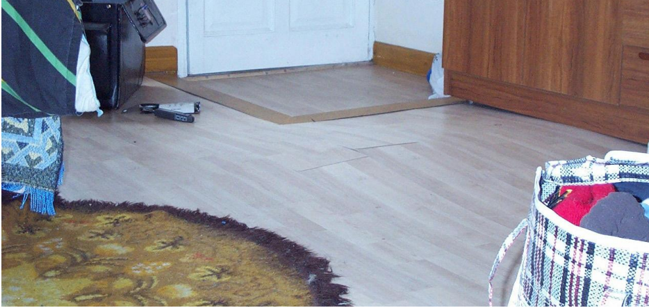
Bulging / distortions
