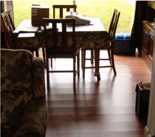
Dishing of laminate floor elements due to lack of vapour barrier (i.e. No DPM over concrete subfloor)
