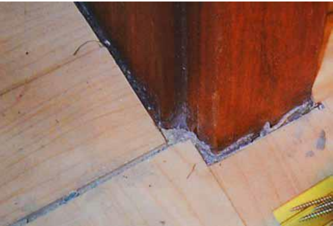
Development of odours (old floor lining was not removed)
