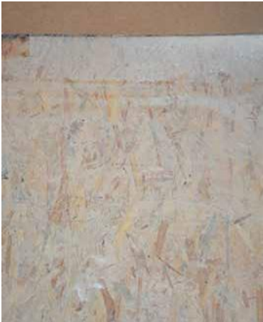
Unsuitable insulation material
