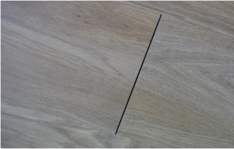
Top joints on laminate flooring elements
