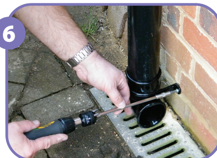
6 Fit the shoe at the bottom of the downpipe so that it directs water into the drain, if required. Secure the joint with a pipe clip.
