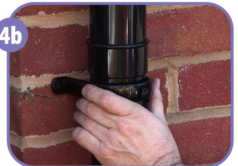
4b Fit the pipe clips to the downpipe and screw them into the wall.
