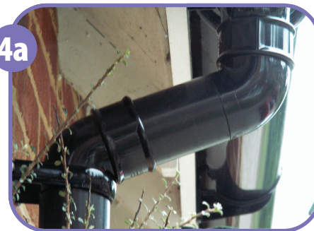
4a Working from the top downwards, install the downpipe. If additional lengths of downpipe are required, join using a socket and pipe clip.
