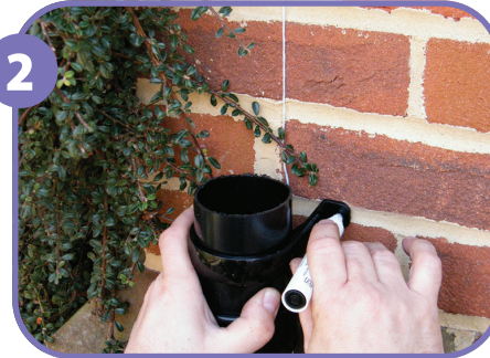
2 Hold a downpipe clip centrally over the line and mark the fixing holes on the wall with a pencil. Repeat down the wall, spacing pipe clips no more than 1.8m apart.
