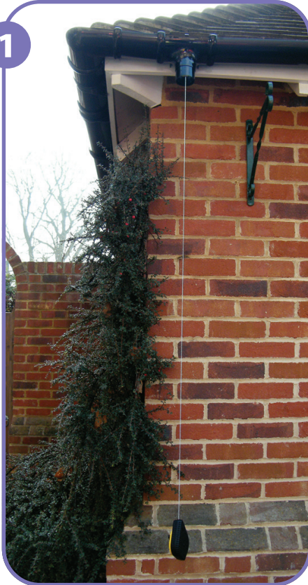
1 Using a plumb line, mark a vertical line on the wall from the outlet to the drain.
