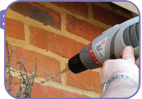
Drill the fixing holes.
