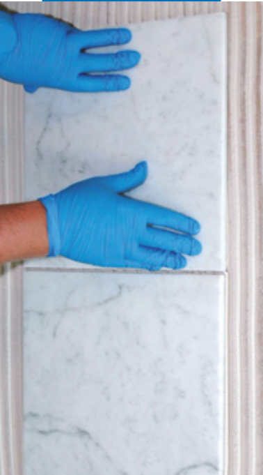
Application of Mapeker Rapid-Set Flex on 15 mm plywood
