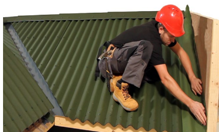
Side wall abutment Metal or preformed proprietary side wall abutments; or Onduband self-adhesive flashing tape are used to seal side wall abutments providing a minimum of 7.5 cm upturn against the wall and dressed over at least one full Onduline corrugation. Complete with a separate wall cover flashing.
