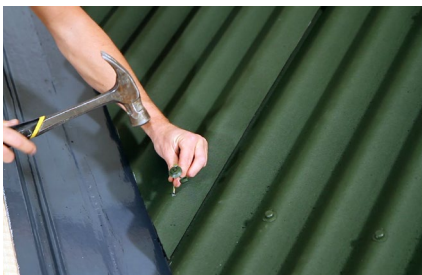
Fixing sheet to valley The sheets are fixed in place allowing for the correct sheet side and end laps. The fixings are secured up the line of the purlin trimming battens.
