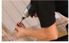
Positioning Onduline Screws Engage screw with a Phillips headed bit (HEX 1/4" PH N02) and position screw centrally through the pre-drilled guide
