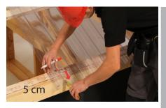
Fixing at the Eaves: Always allow for a 5cm sheet overhang from the fascia. This provides a water shed point for rainwater into the rainwater collection system.
