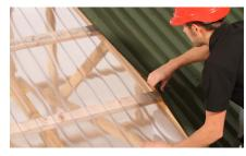
Fixing PC sheets in Onduline roof: When fixing PC sheets with Onduline Bitumen Sheets always lap the Bitumen Sheet onto the PC sheet. Never lap the PC sheet onto the darker surface.
