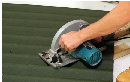
Cutting sheet Remove the sheets from the roof supporting either side of the required cut line, then use a mechanical saw to cut the sheets as required.
