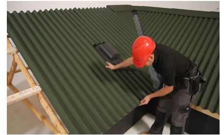
Onduline verge pieces The ventilators are fixed between the purlins. The apron is lapped over the lower sheet, with the integral side and back gutter aprons being lapped by next.
