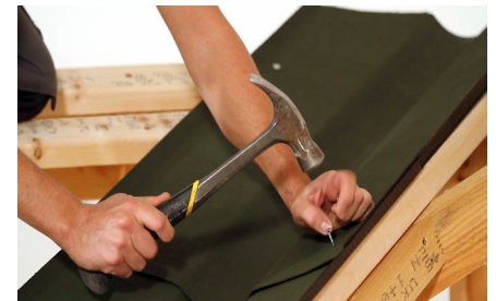
Fixing valley lining The Onduline units are secured to the purlin trimming battens by nailings at 20cm centres up the line of the gutter.
