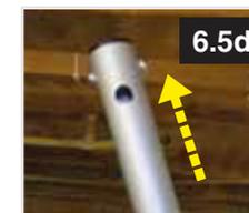
Repeat the same setting on the right-hand top stile from step 6.2. Note that this stile must be rotated 90 degrees and 180 degrees counter clockwise for 150 and 300mm extensions respectively.
