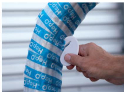
Figure 21: Always protect pipe ends
