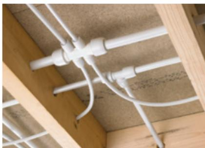
The exceptional flexibility of Hep<sub>2</sub>O pipe removes most of these restrictions by allowing pipe to be easily curved and 'cabled' through drilled joists, or I-beams which means:
