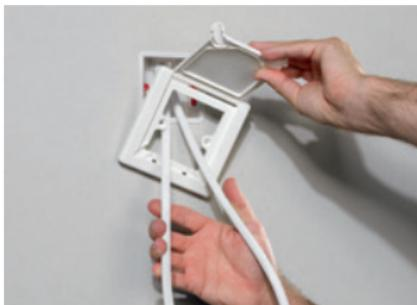
2. Fit cover plate which provides an airtight seal when closed
